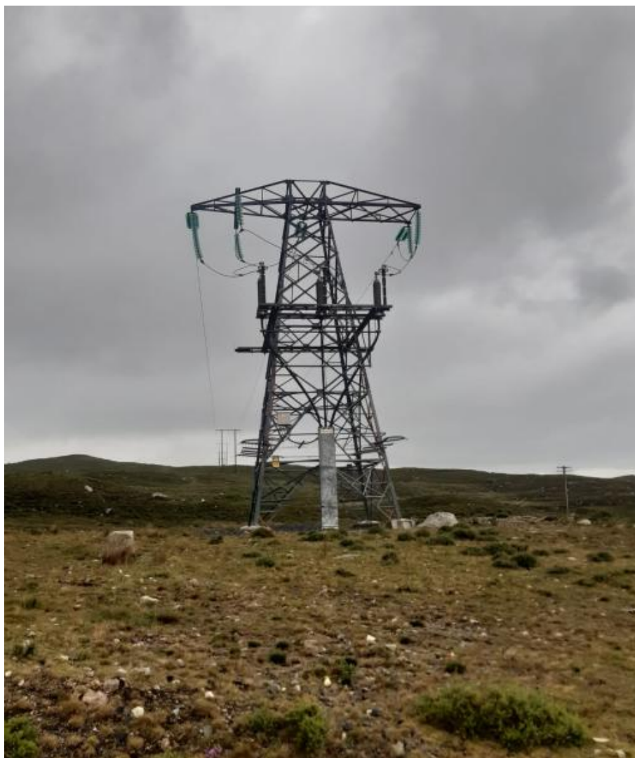
Plate 3-5: Steel Lattice Tower Complete. Source: Applicant, Ardderroo Wind Farm, Co. Galway.
