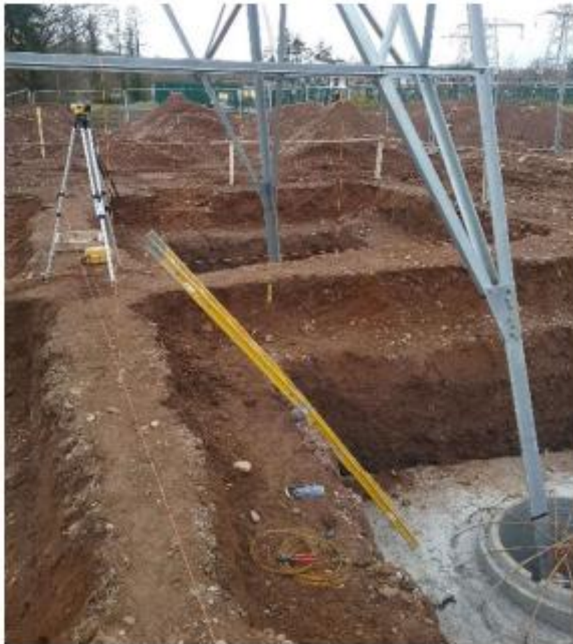
Plate 3-4: Standard 110kV mast foundation excavation. Source: Tli Group
