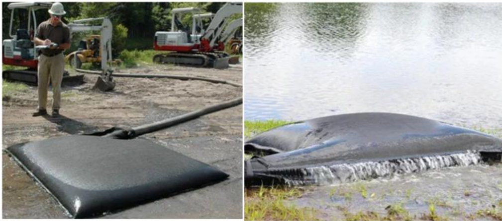
Plate 3-2: Example of Silt Bags in use. Source: Ultra-Dewatering Bags® Oil & Sediment Model | Contain Sediment and Oil — Consolidated Containment
